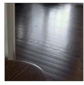
The center of the pieces of flooring appears to be higher than the edges.
