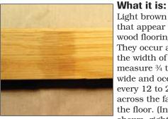
Light brown marks that appear on the wood flooring surface. They occur across the width of the strip. measure <sup>3</sup>/<sub>4</sub> to 1 inch wide and occur about every 12 to 24 inches across the face of the floor. (In photo shown, right side of
